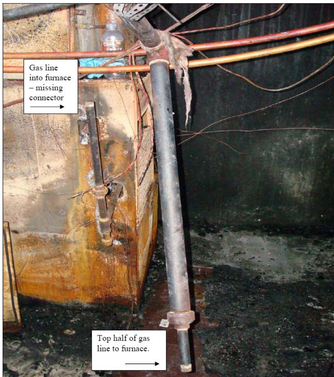
Photo 3. Gas line to furnace. Part connecting top line (end near floor) and line into furnace is missing. (NIOSH photo)
