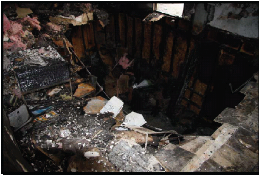
Figure 5: Interior photo of the collapsed area and flooring system. (Colerain Fire & EMS)
