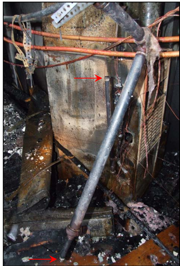
Figure 30: Exposed male ends of the building's furnace natural gas supply piping.
