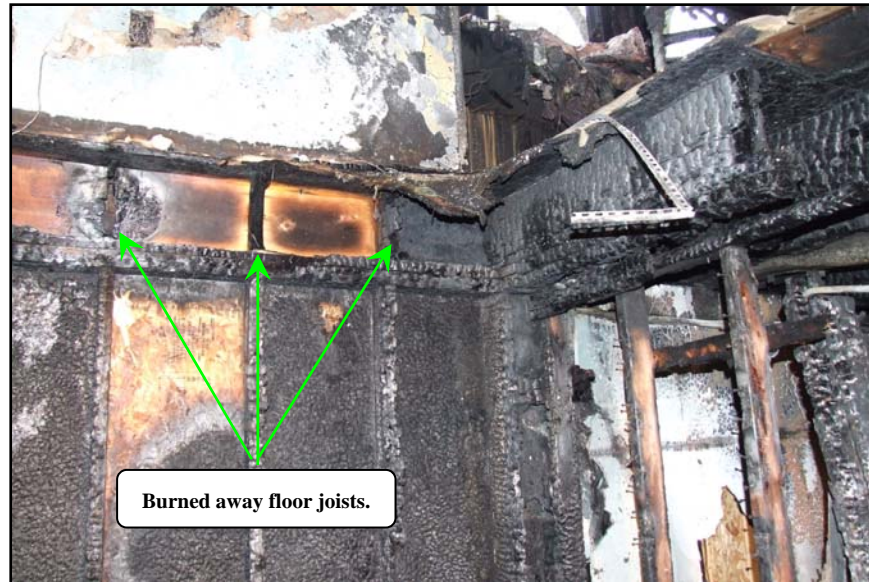
Figure 25: Extensive burn damage to floor joists.
