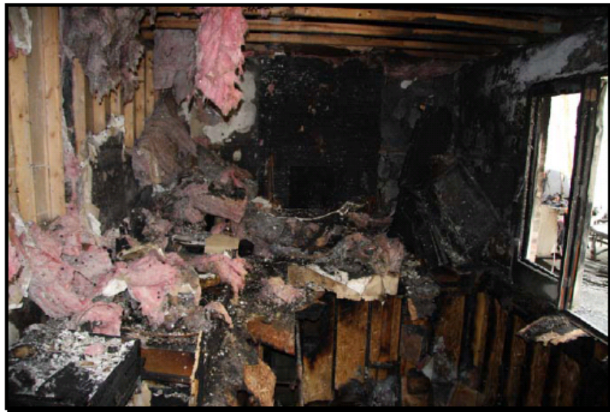
Figure6: Expanded interior photo of the collapsed area and flooring system. (Colerain Fire & EMS)
