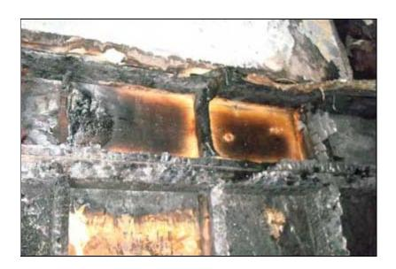
Photo 6. Burned away floor joists above the small cedar closet along the C-side wall.
