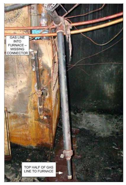
Photo 3. Gas line to furnace. Part connecting top line (end near floor) and line into furnace is missing. (NIOSH photo)
